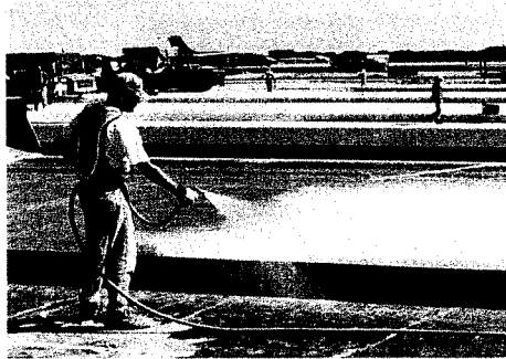
Fig. 12-8. Liquid membrane-forming curing compounds should be applied with uniform and adequate coverage over the entire surface and edges for effective, extended curing of concrete. (69975)
