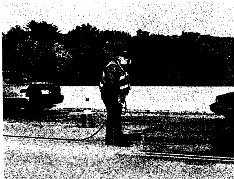
Fig 12-12. Penetrating sealers help protect reinforcing steel in bridge decks from corrosion due to chloride infiltration without reducing surface friction. (69976)
