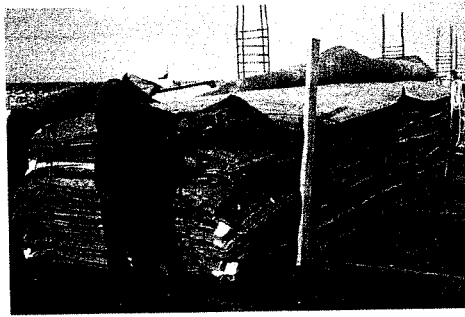
Fig. 14-19. Stack of insulating blankets. These blankets trap heat and moisture in the concrete, providing beneficial curing. (43460)
